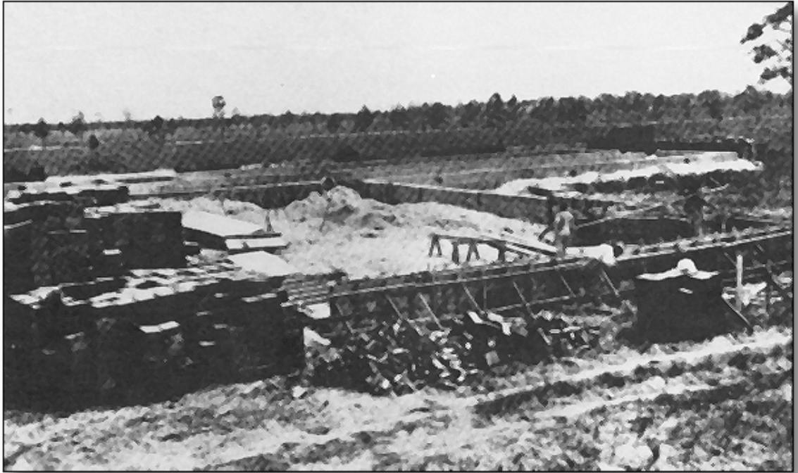
$200,000 school under construction near the Tamiami Trail Entrance of Edison Park.
